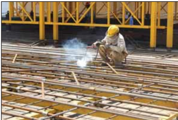
Fig. 2.15. Welding of reinforcement cage
