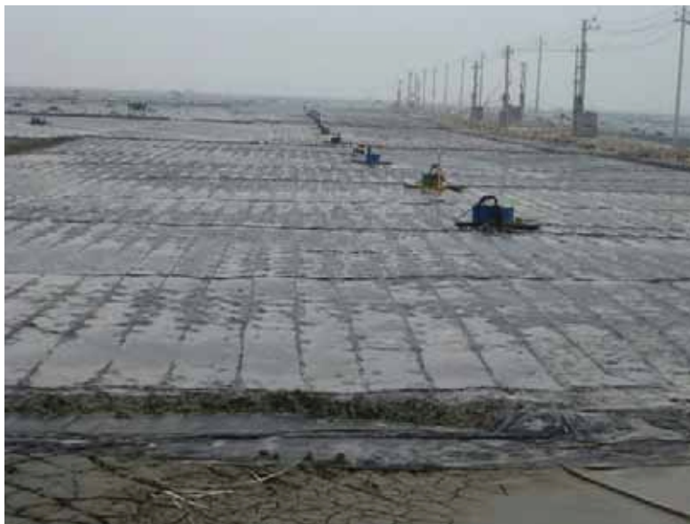
Fig. 8.9. Multiple smaller water-jet vacuum pumps used on another project site (photo taken by Jie Han in 2010)
