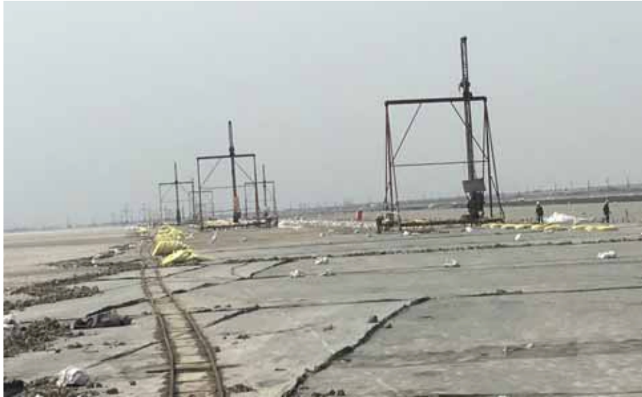
Fig. 8.12. Light weight wick drain installation rigs over the very soft reclaimed land
