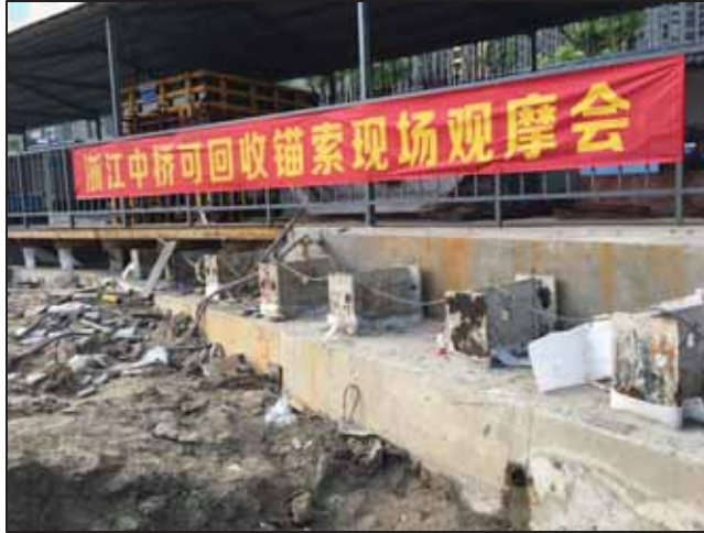
Fig. 4.8. Reusable wide flange beams and detachable anchors in an earth retaining wall in Xiaoshan Sci-Tech City South District, Hangzhou, Zhejiang Province.
