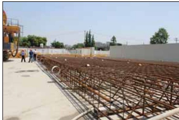
Fig. 2.16. Completed reinforcement cage
