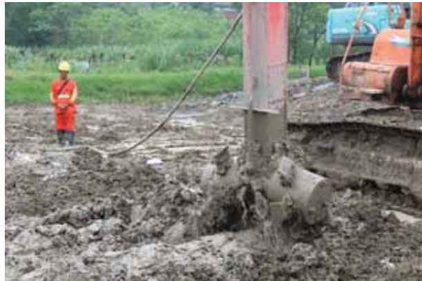
(c) Grout injection from the mixing tool
