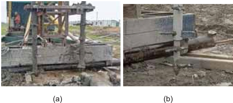
Fig. 5.2. DSM Mixing Tools (single and bi-directional rotation types)
