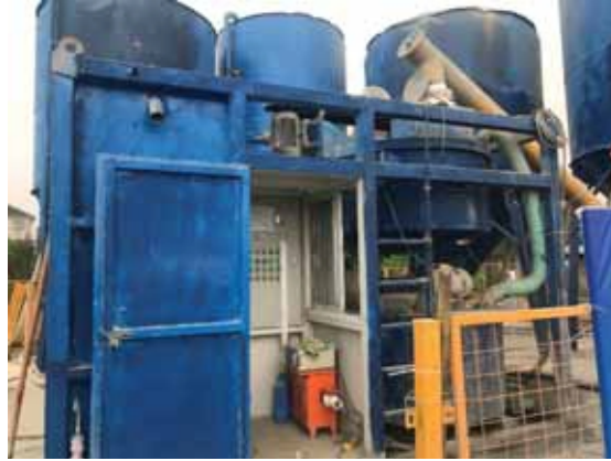
Fig. 6.2. The binder or grout supply system
