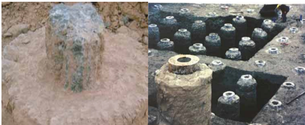
Figure 11.12. Examples of composite columns in the field (Zheng, 2018)
