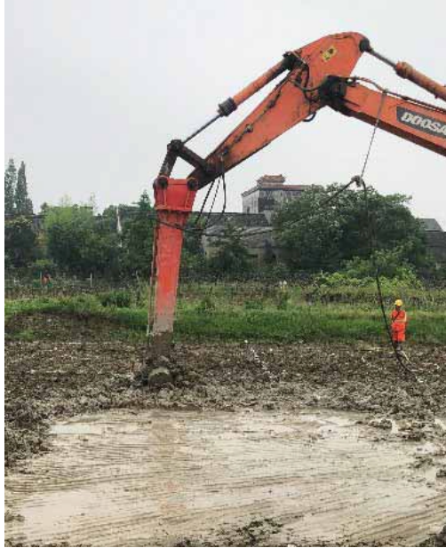
Fig. 6.5. Final surface of shallow soil mixing prior to curing
