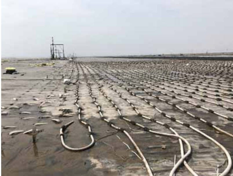
Fig. 8.6 PVD Installation and connection to horizontal vacuum tubes
