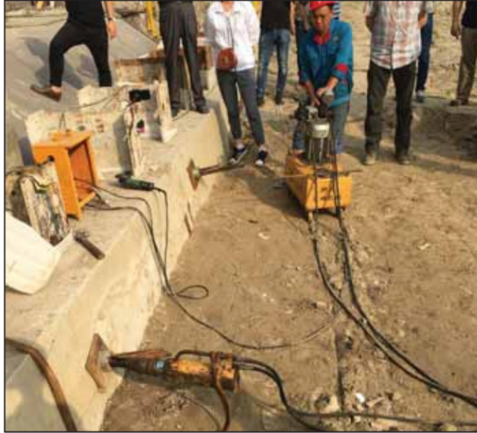
Fig. 4.4. A mono jack pulling the reclaiming cable to release the locking wedges.
