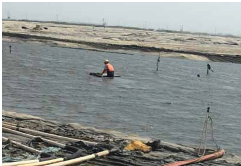
Fig. 8.11 Detect and repair leakage liner
