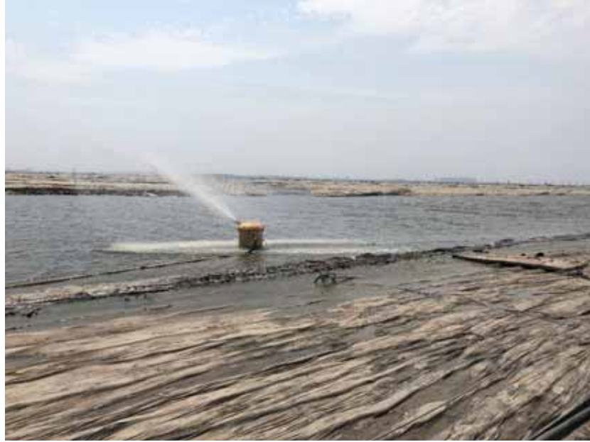
Fig. 8.10. Area under vacuum preloading
