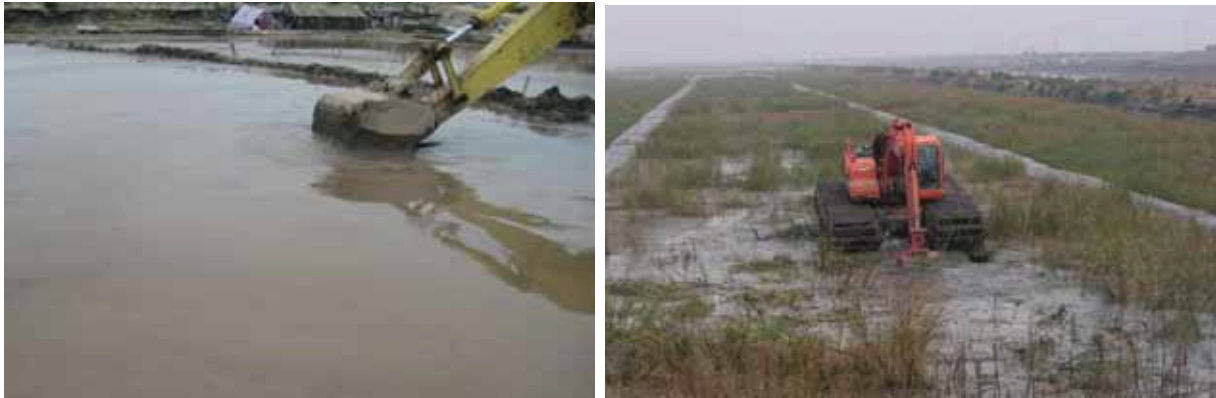
Fig. 3.2. Disturbance of hydraulic fill to a denser state (source: Shanghai GeoHarbour Co.)
