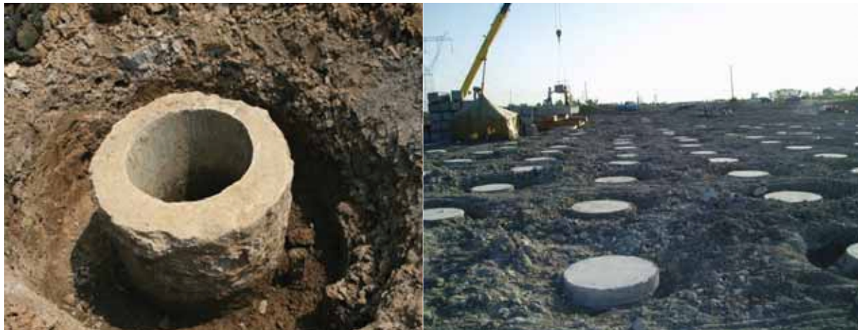
(a) Exposed pipe pile
